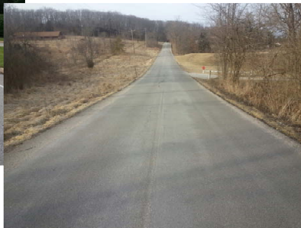
Fog Seals perform well on pavements in better condition.
