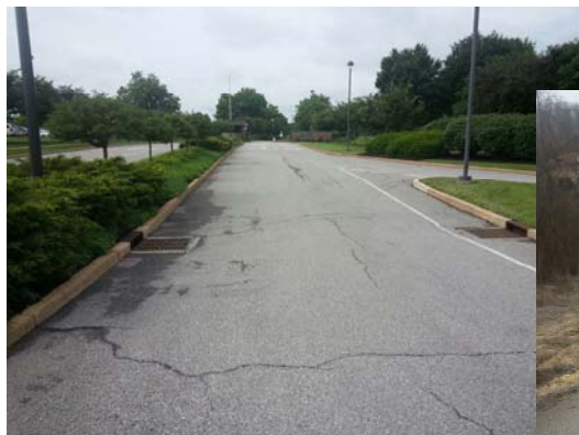
An aggregate based system will fill in surface voids and raveled areas.
