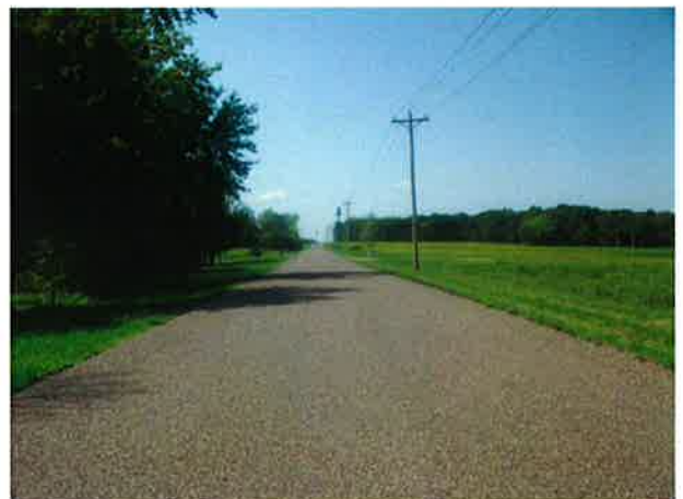
A 3/8" trap rock CHFRS2P chip seal placed in 2012 in Lincoln County
