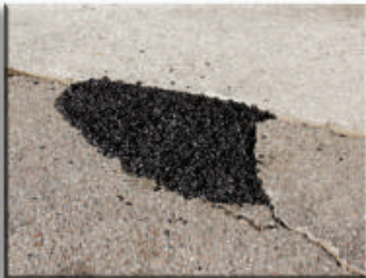
Spread HP in two inch (2") increments, outward to each edge of the area to be repaired.
