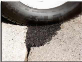
Compact or tamp into place. Open to traffic immediately. It's that simple!
