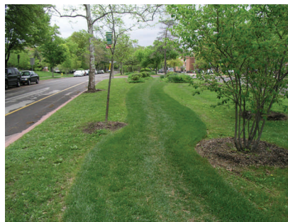
Soil and sod were placed over the Grasspave2 grid.
