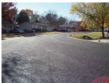
GSB-88 is applied to a recently constructed chip seal.
