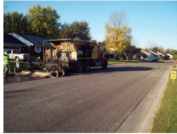
Microsurfacing is placed on a chip sealed surface.
