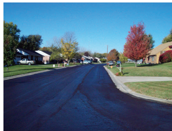
The completed project.
