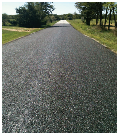
GSB-88 applied to a limestone chipseal
