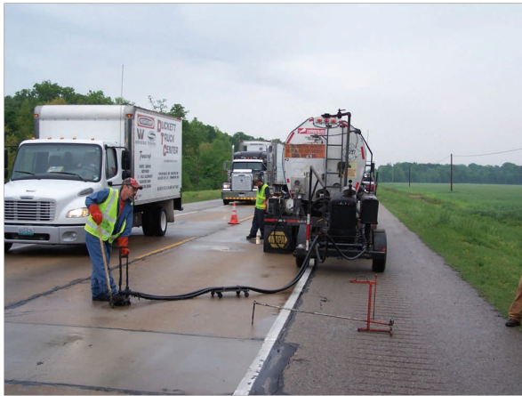
The asphalt undersealing operation
