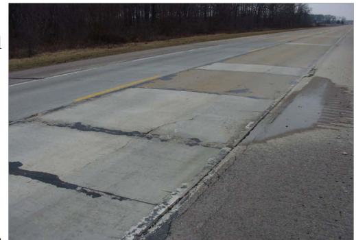
Water Pumping from the subgrade of Rte. 67 before repairs
